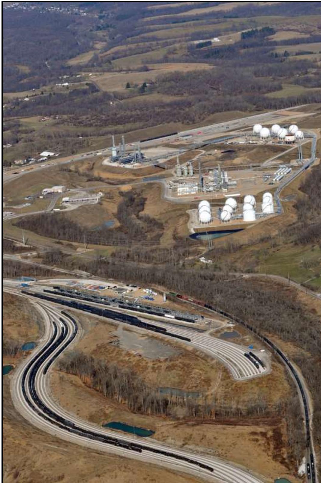
Figure 12 – One of several major gas processing plants upwind in eastern Ohio CADIZ, OHIO
