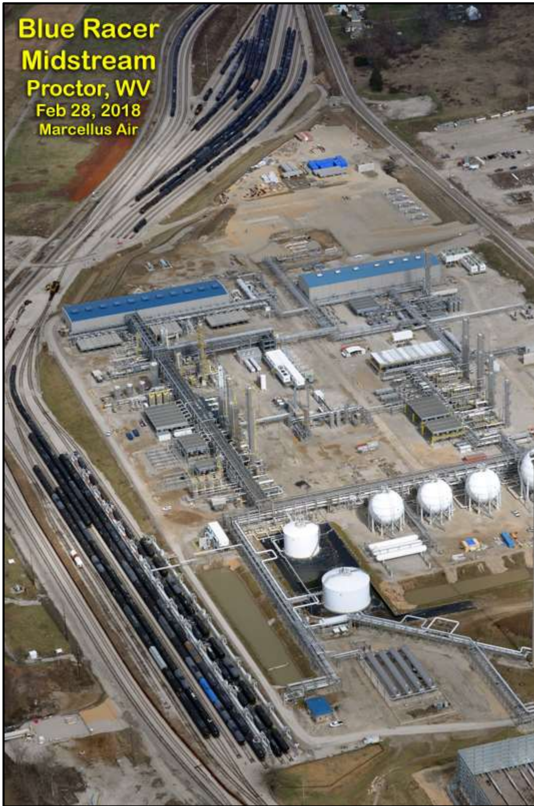
Figure 11 – One of several major gas processing plants in northern West Virginia
