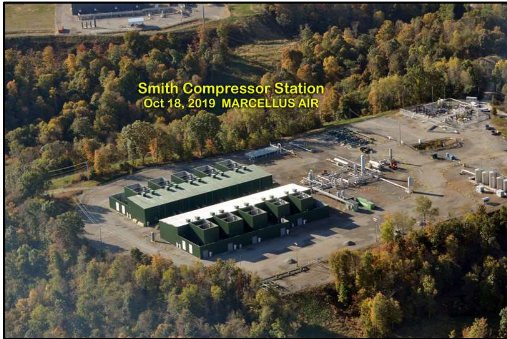
Figure 5 – Huge compressor station in Washington County, PA
